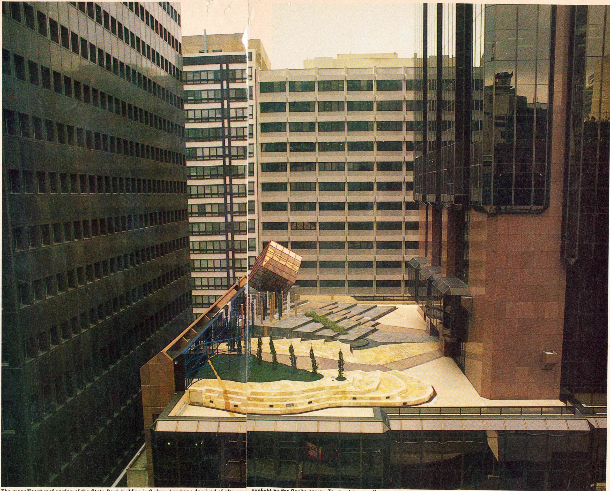
The magnificent roof garden of the State Bank building in Sydney has been deprived of afternoon sunlight by the Capita tower. The bank is an effort to recapture the romance of the 1930s US skyscrapers.
